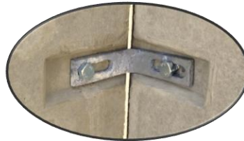
Detail 1 Eckverbinding
