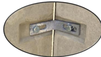
Detail 1 hoekverbinding
