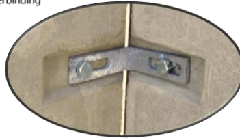
Detail 1 hoekverbinding
