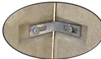
Detail 1 Eckverbinding
